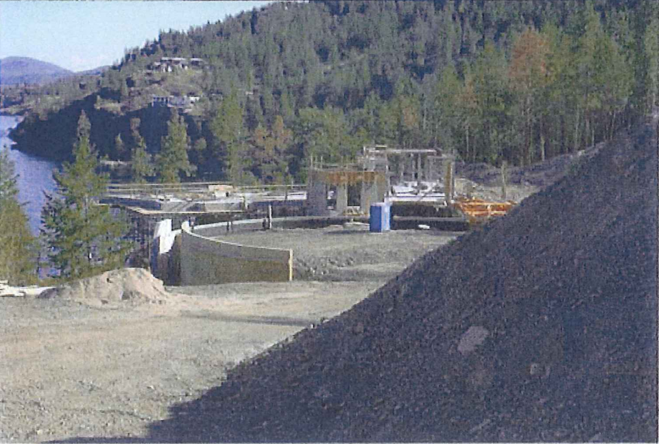
10-180 Sheerwater Court Guest House Site Photos
